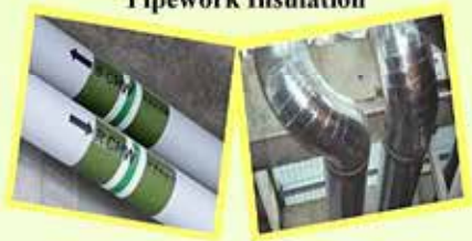
Chilled Water Pipework Insulation
